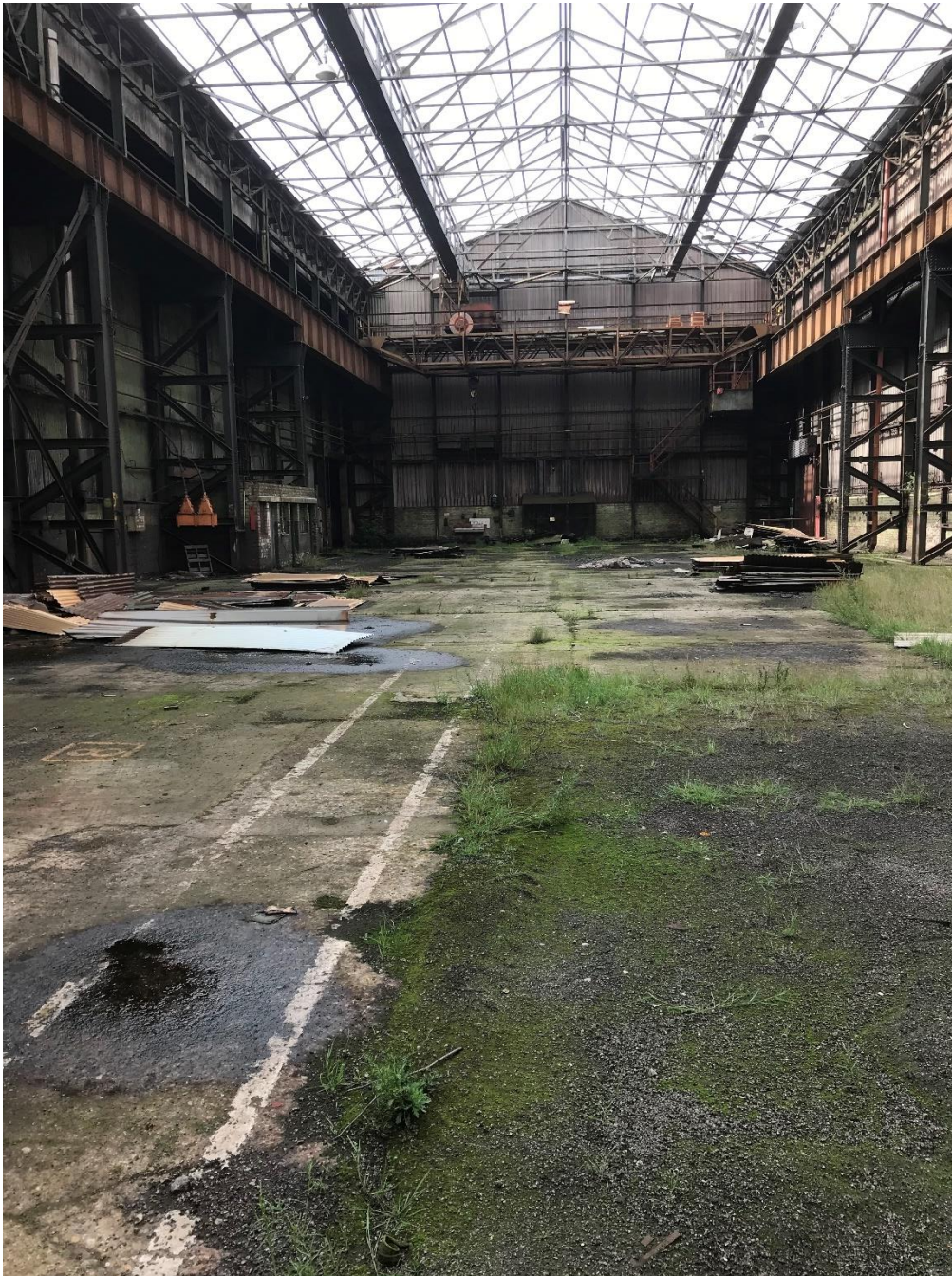
Photograph 4 – Interior of structure B1a
