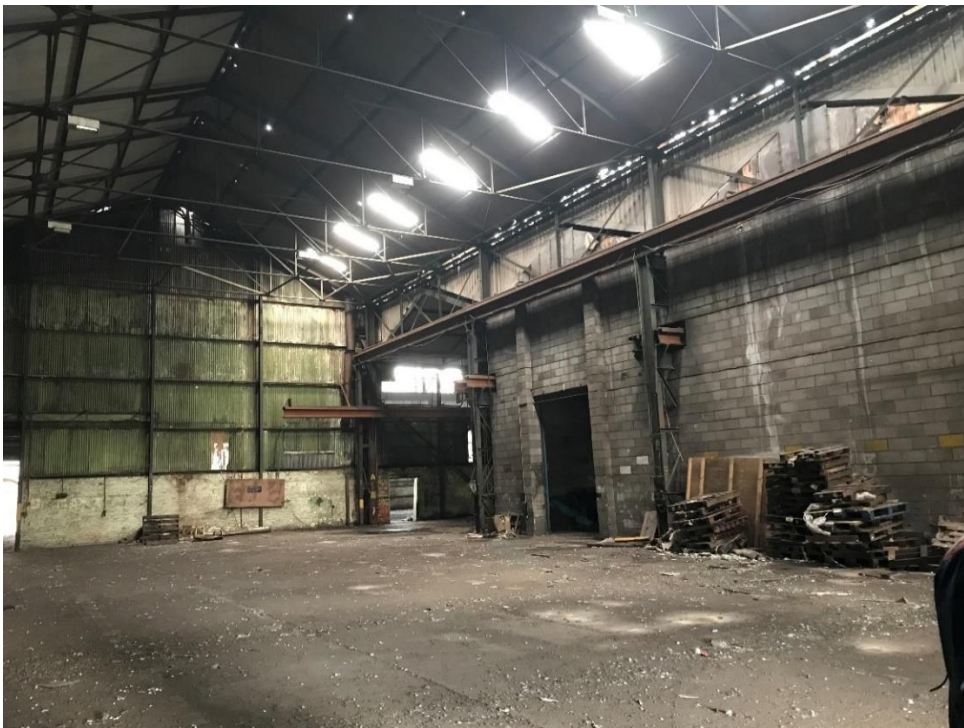
Photograph 2 – Interior of structure B1a
