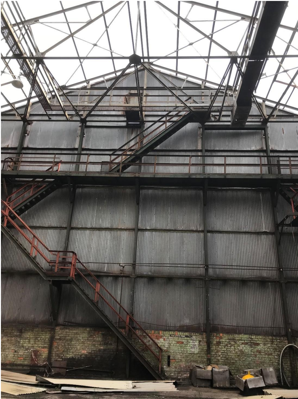
Photograph 3 – Interior of structure B1a
